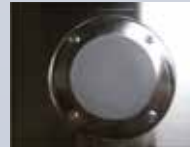
Port for CO 2 fire extinguisher
